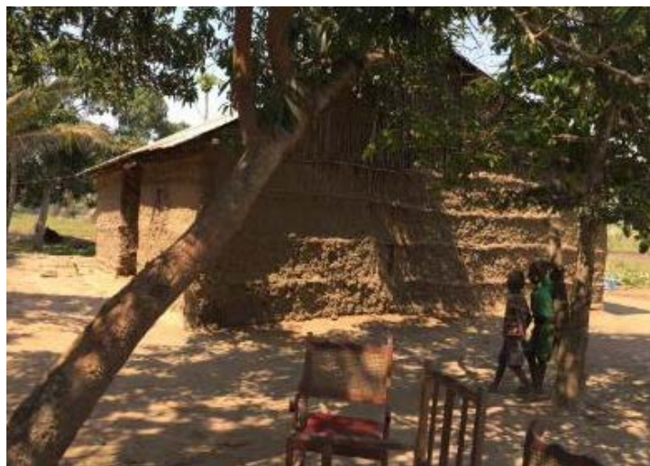
FIGURE 2. A Typical Mud and Mangrove Poles House in Mirazane
